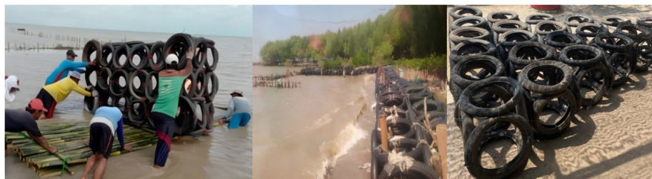
Figure 4. APPOSTRAPS technological innovation utilizes waste tires to overcome abrasion.
