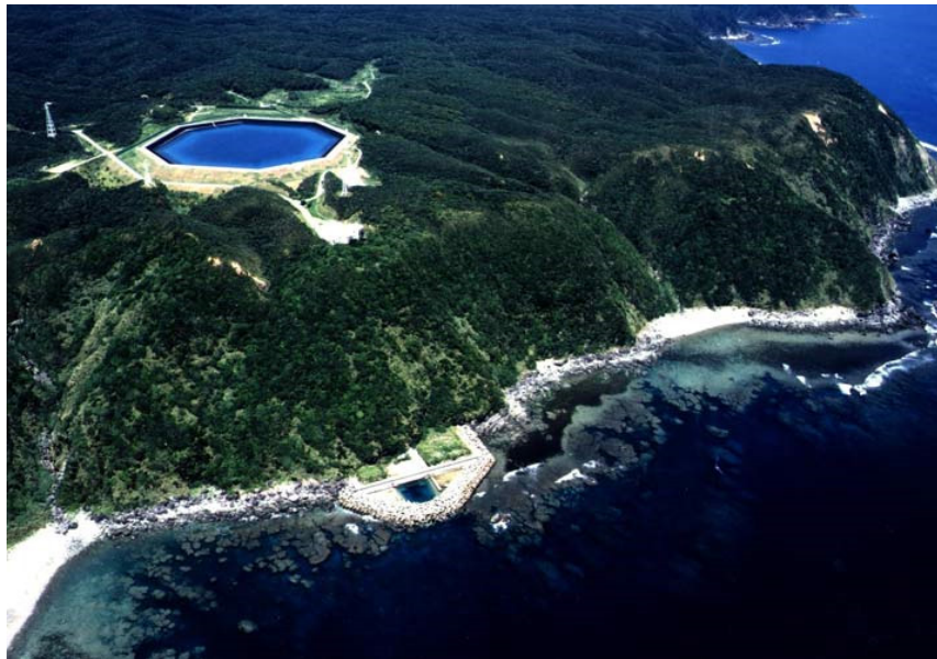
Figure 2. Okinawa Yanbaru coastal PHEs plant, 30 MW capacity.
