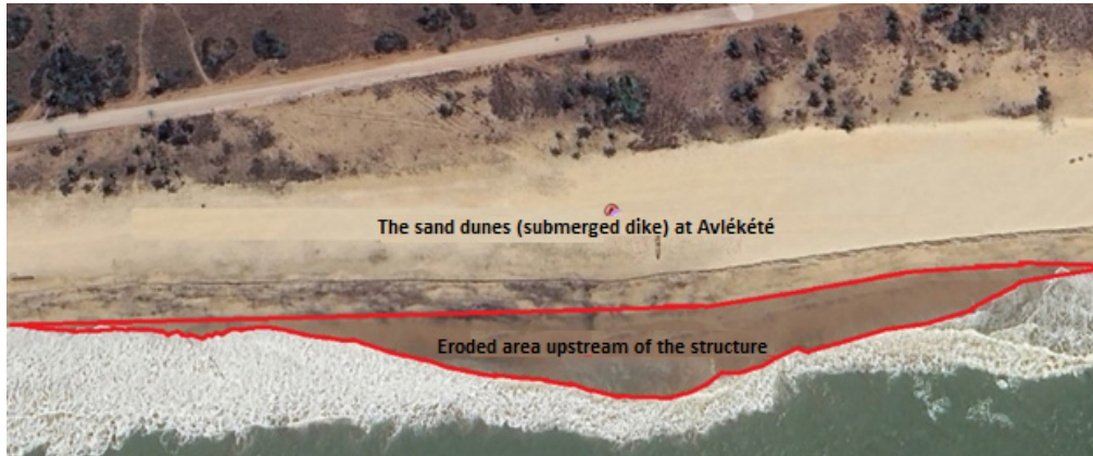
Figure 1. Submerged Avlékété Breakwater with Upstream Erosion in 2025.
