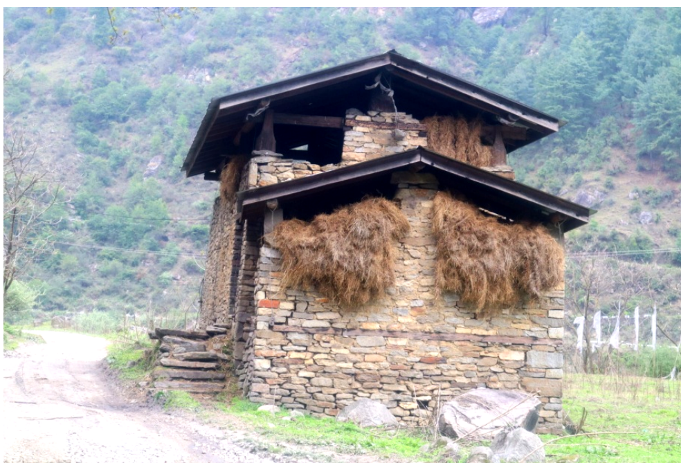
Figure 1. Dry fodder stored in the storage compartment build in a stone house owned by a yak herder in zemithang valley of tawang district.
