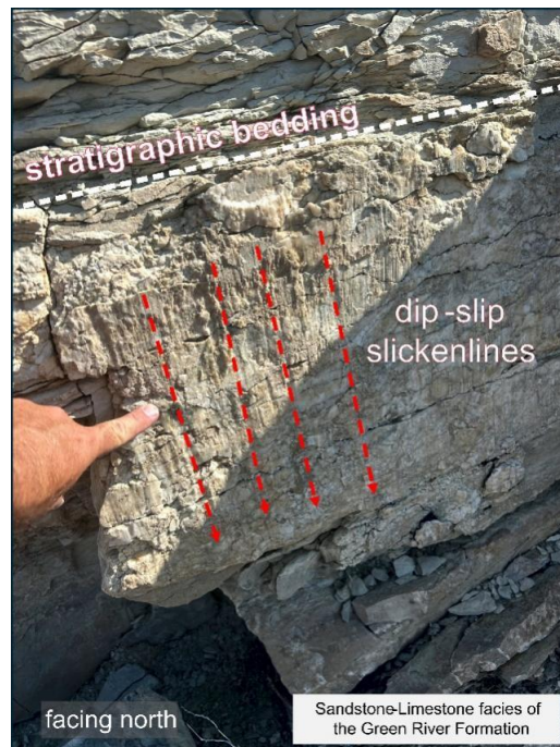
Figure 13. Near-vertical normal fault bounding the DG horsts.
