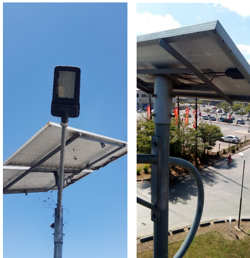
Figure 1. Fixed System of Solar Panels to Ensure Power Output is Maximized in Lusaka.
